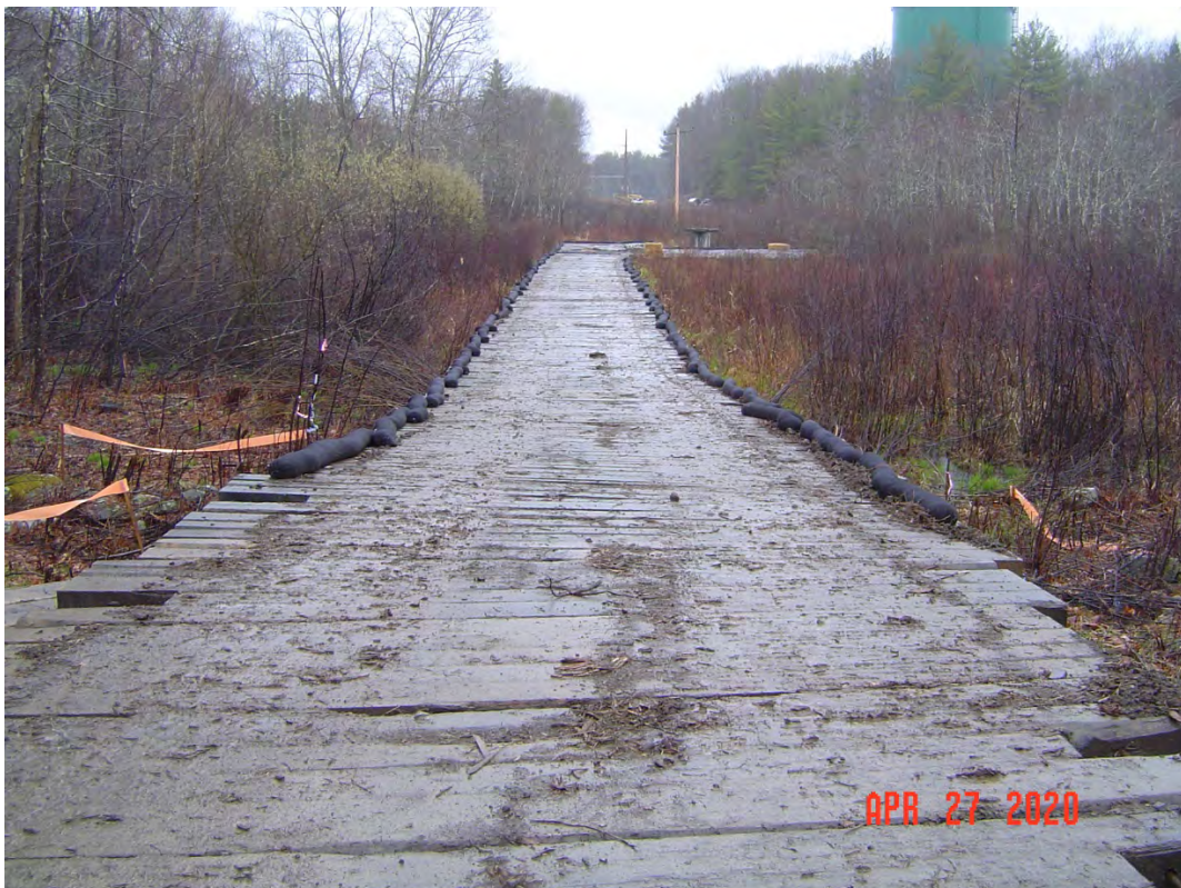
Fig 6: Access road through wetland DW41 to Str. 35 work area. Viewing northeast. (04-27-20).
