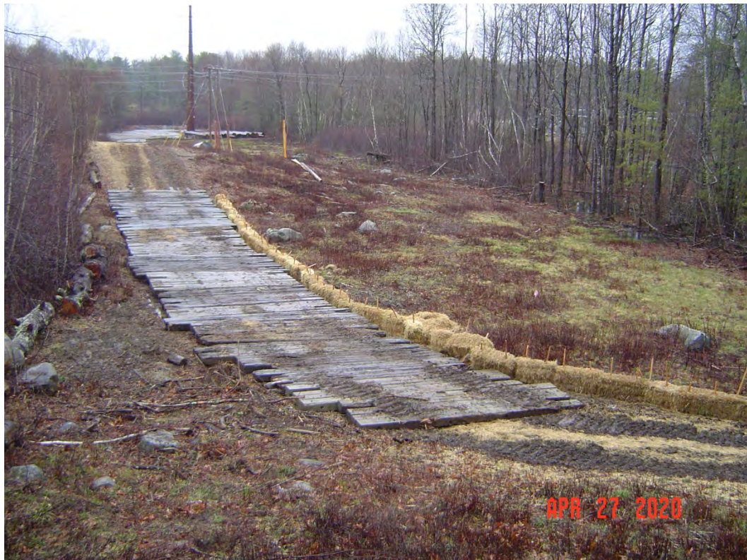
Fig 8: Access road between Strs 46-47, next to wetland DW56. Viewing southwest. (04-27-20).
