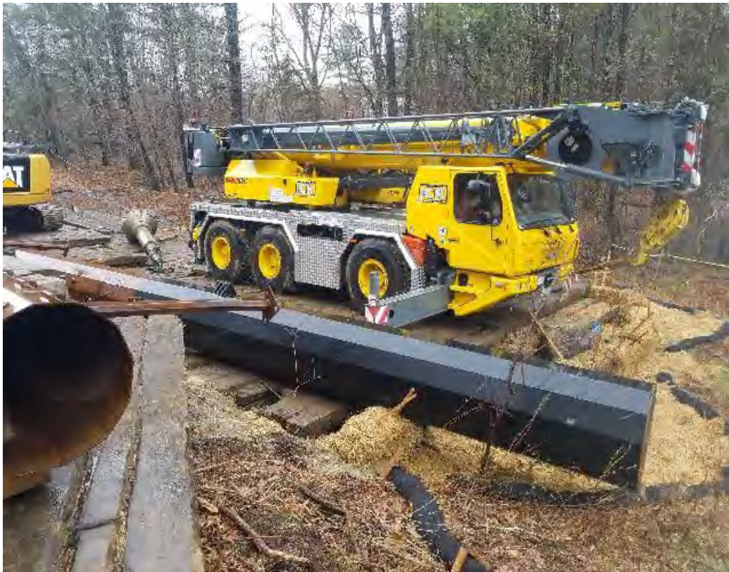
Fig 4: Str. 89 work area. Viewing northeast. (04-27-20).
