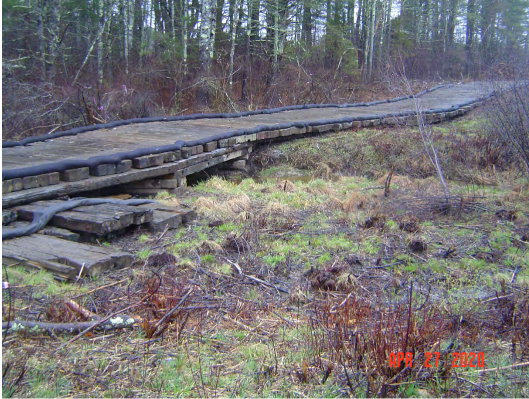
Fig 9: Access road bridged over stream DS60, in wetland DW58. Viewing southeast. (04-27-20).
