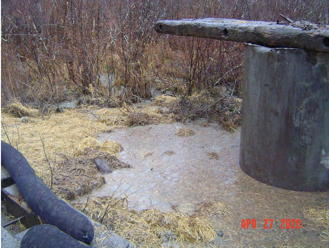
Fig 7: Hard can set in wetland DW41 for Str. 35. Viewing north. (04-27-20).
